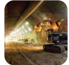
Tunnels, Pilling & Post Tensioning
